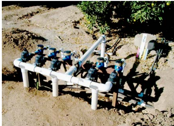
Block 13 at UCR Citrus Research Center and Agricultural Experiment Station - controls for applying the partial root zone drying (PRD) and reduced conventional (CI-RR) and control irrigation (CI) treatments to 'Washington' navel orange trees.
